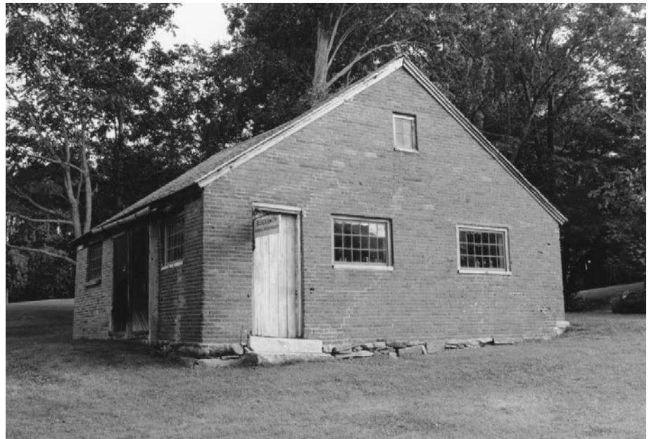
The Ashbel Goodenough Blacksmith Shop
